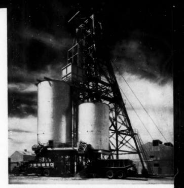
**HEADFRAME** at five-compartment Palo Verde shaft is 120 feet high with 500-ton ore and 250-ton waste bins attached.
